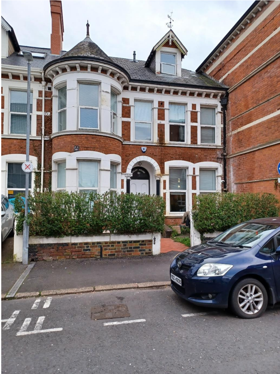
Appendix 1 – External Photographs and Location Map – 6 Sandhurst Road, Belfast, BT7 1PW
